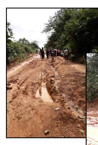
This is but a tiny sample of the mayhem we've experienced this rainy season as our road is washed out in several places. This mud is especially slick and builds up on tires making it very difficult to control the vehicle. Passengers walk around these mud traps reboarding their vehicle on the other side.
